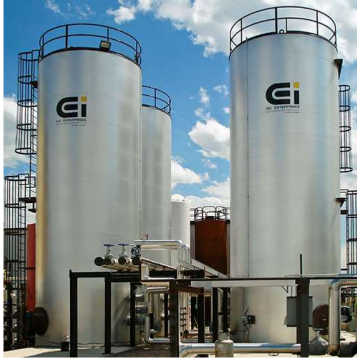
Figure 2-10. Vertical storage tanks (CEI Enterprises, 2008)
